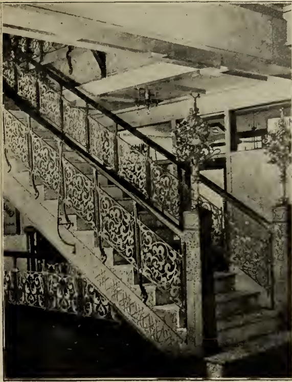
A.—STAIRWAY, MONADNOCK BUILDING, CHICAGO. Cast Aluminium.
